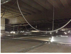
Fig. 5. Dropped Ceiling Cavity
