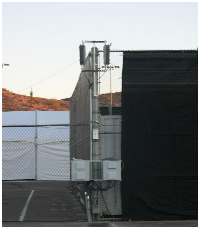
Figure 7: Due to the small form factor, Small Cells were installed on existing infrastructures; existing fence in this example
