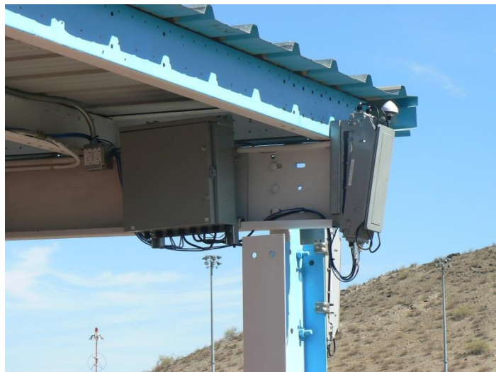
Figure 6: Airspan Airsynergy 2000 with the front mounted 11 dBi, 65 degrees horizontal beamwidth, antenna.
