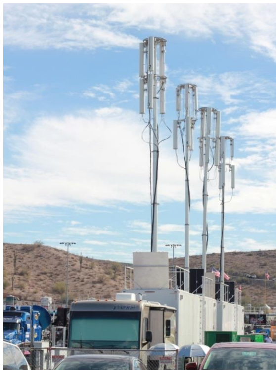
Figure 8: In NASCAR venues, coverage and capacity is typically provided by rolling in Cell-on-Wheel.
