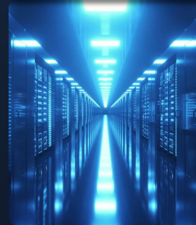
WIRELESS DATA CENTER
